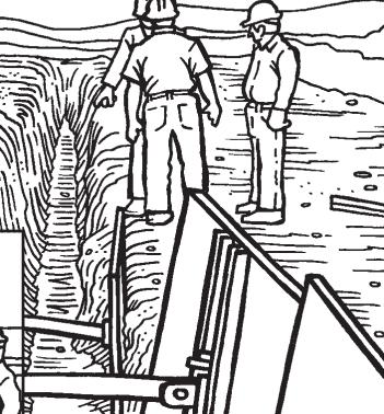
CORRECT - Barricade correctly in place to keep personnel from getting too close to an open trench
